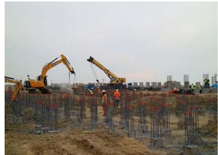
3GP Site Preparation Progress
