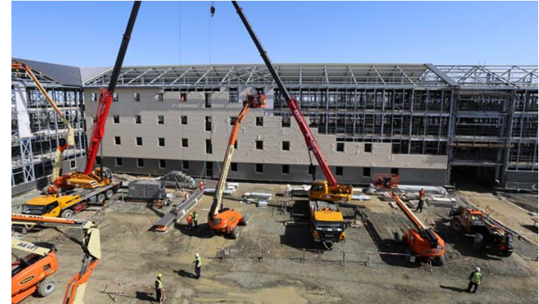
Orken Village construction progress
